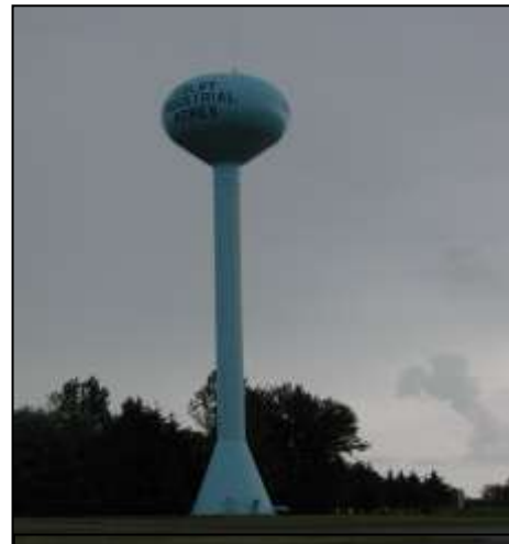
The City of Colby Industrial Acres (Park) contains public water and sewer infrastructure.
