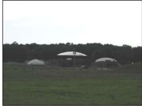
Colby wastewater treatment plant.
