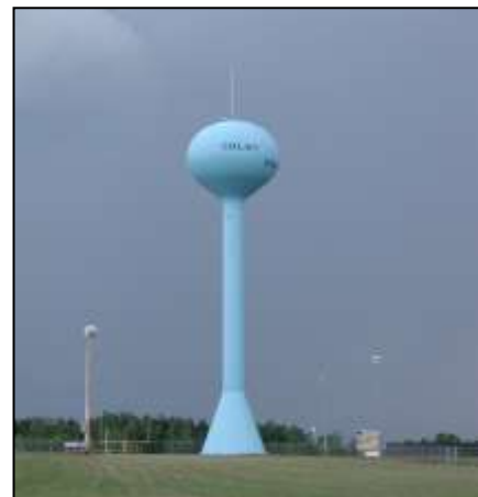
Colby water tower.
